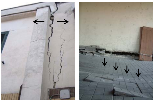
Figure 2. Effects on buildings induced by subsidence: examples of structural (left) and non-structural (right) damages.
