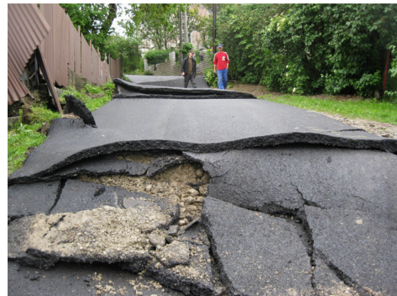
Figure 1. Local communication destroyed by the Nizna Mysla landslide [1]
